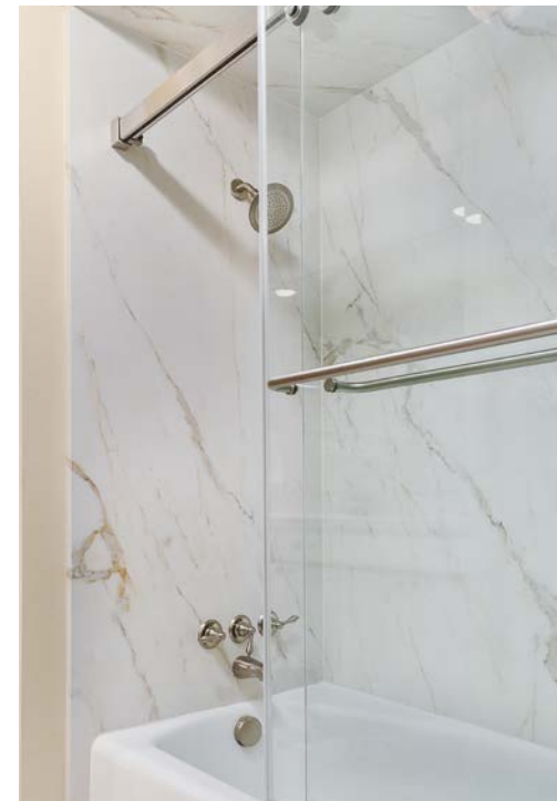
Porcelain slab over existing tile – no tear out
