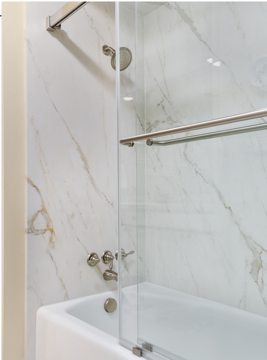
Porcelain slab over existing tile – no tear out
